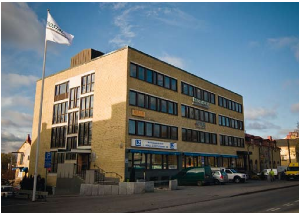
Brostaden's main office on Bolidenvägen is GreenBuilding classified.
